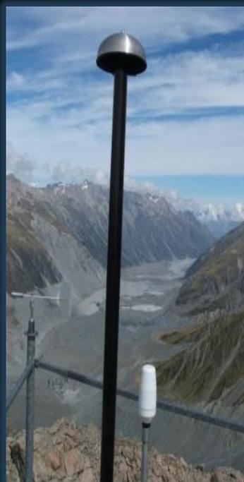
*The DYNASPHERE air terminal mounted at the top of an insulated mast through which the discharge current is safely conveyed to the ground.*
